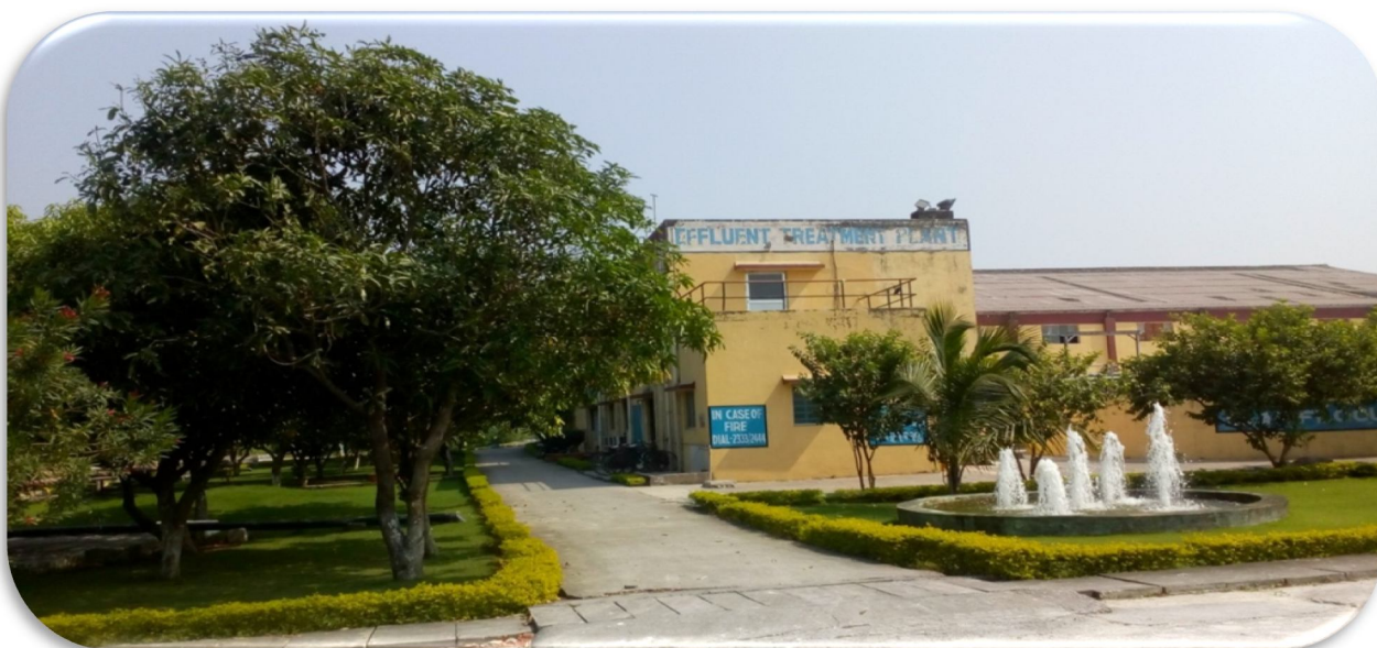
Plant inside view
