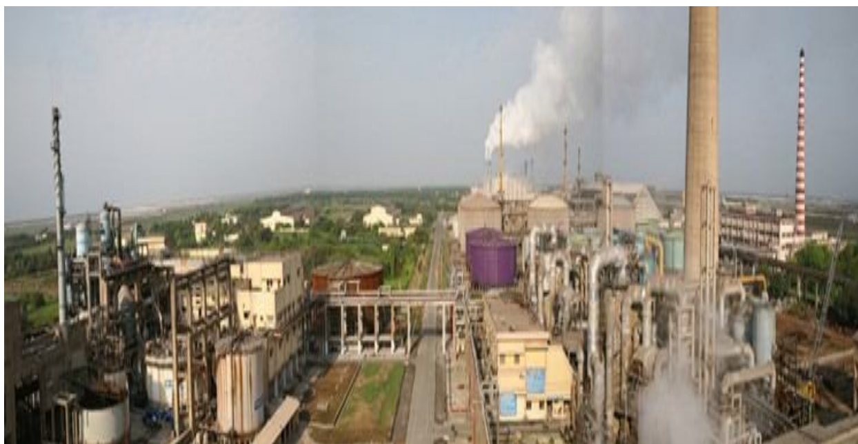
Plant inside view
