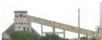
Concrete Enclosures For Conveyor Belts
