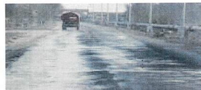
Truck Mounted Water Sprinkler
