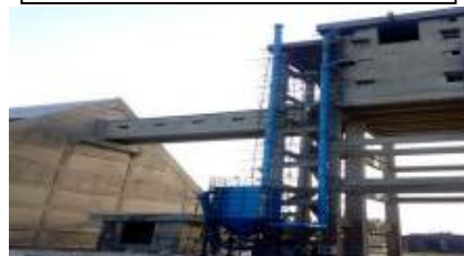
Bag Filter Installed at Jetty
