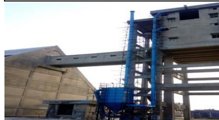
Bag Filter Installed at Jetty
