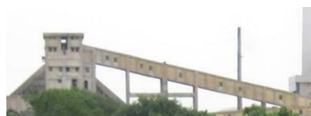
Concrete Enclosures For Conveyor Belts
