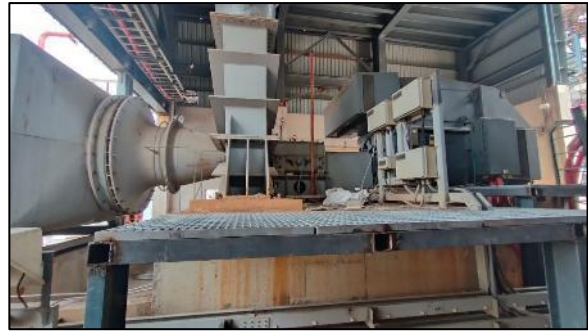
Installation of blower
