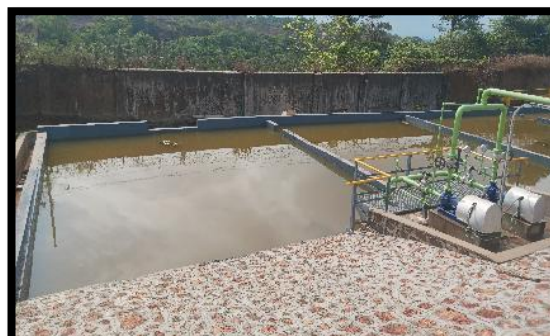
Catchment Pit – Goa facility
